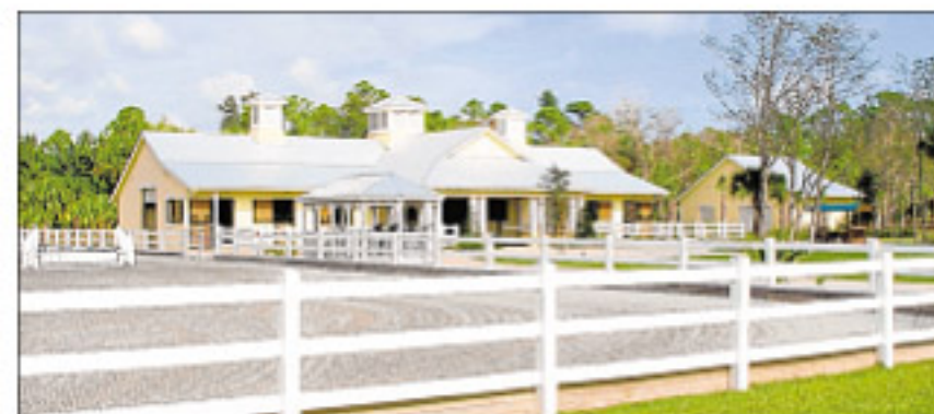
Designed by Affiniti Architects and built by Cribb Construction, this barn's open design and the construction of the stalls allows for natural cooling, as well as the ability to be completely closed in poor weather. The hurricane-resistant barn features eight stalls with individual run-out areas, a fly-spray system, swinging feeders and an automatic watering system for convenience and safety, a groom's apartment, feed room and two wash stalls.
